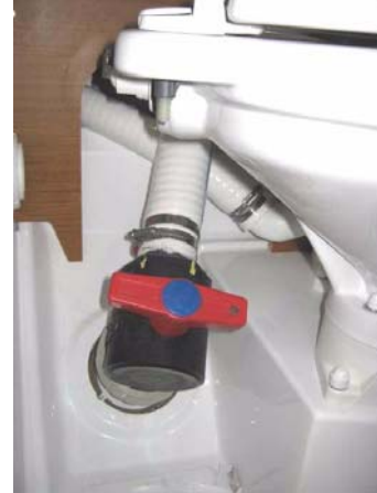
WC evacuation gate valve to sea
