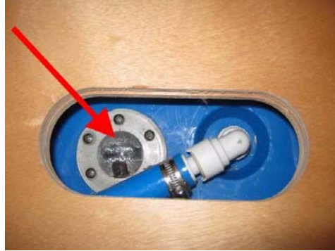
Gauge (located directly on the tank)
