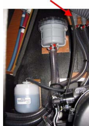
Location: Engine compartment
