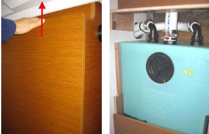
Black water tank Location: Head version Capacity: 80A
